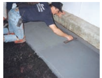
Application by hand trowel
