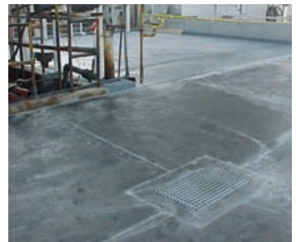
Finished flooring project
