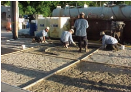
Constructing forms after surface preparation Photos courtesy of the authors
