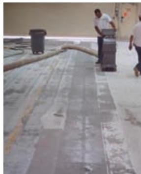
Surface Preparation (first of two passes)
