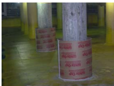
Figure 3. The forms placed around the column.
