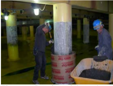
Figure 4. Pouring of the polymer concrete.
