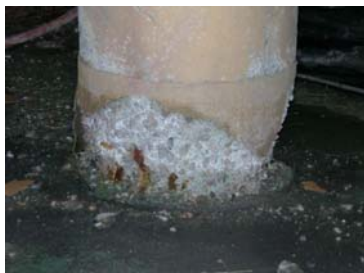
Figure 1. Column Degradation.
