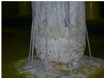
Figure 2. Stainless steel rebar bent and grouted into the channels.
