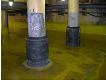
Figure 5. Columns after removal of forms.
