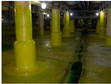
Figure 9. Completed column repair.
