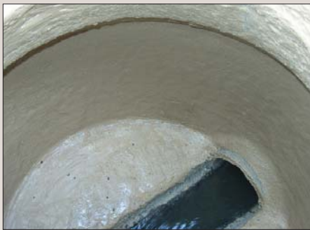
An example of a manhole rehabbed using Sauereisen's epoxy liner.
