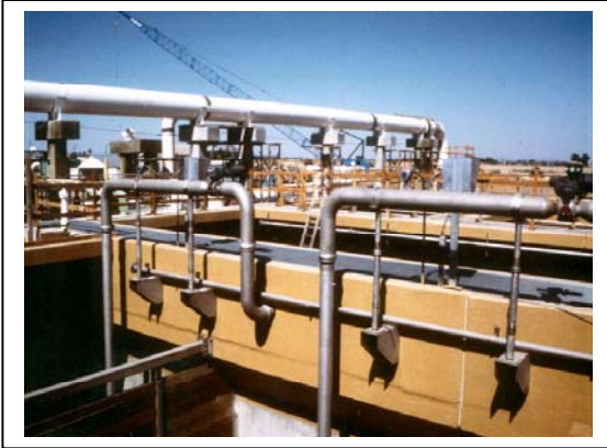
Completed SewerGard No. 210T lining installation
