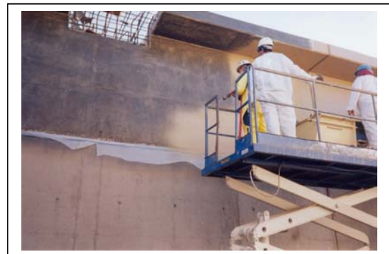
Vertical surfaces were easily lined with the Trowel version of the SewerGard product.
