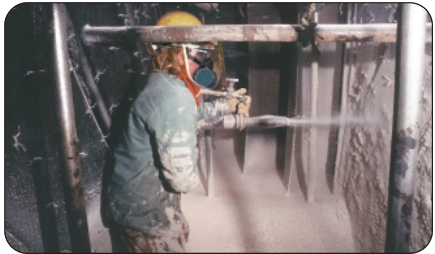
Gunited refractories are a solution where aggressive acids are combined with high temperatures.
