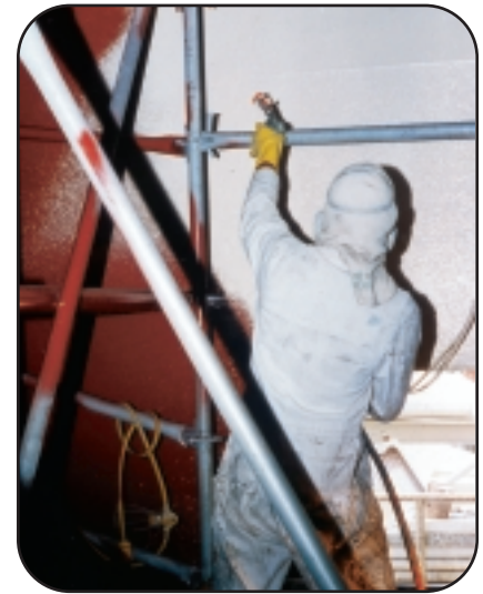
Applying Vinyl Ester FibreLine by spray.
