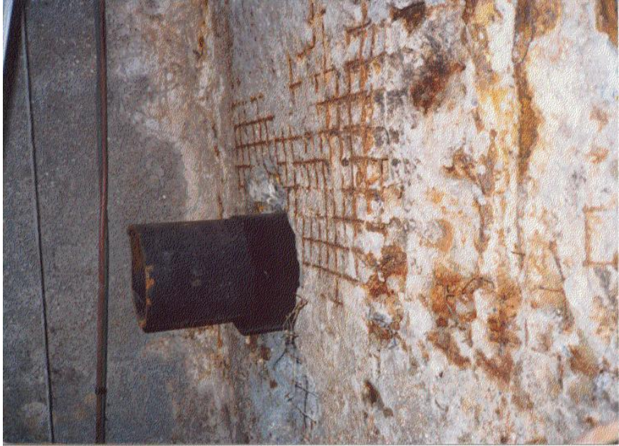
Figure 4. Lift Station Prior to Rehabilitation.
