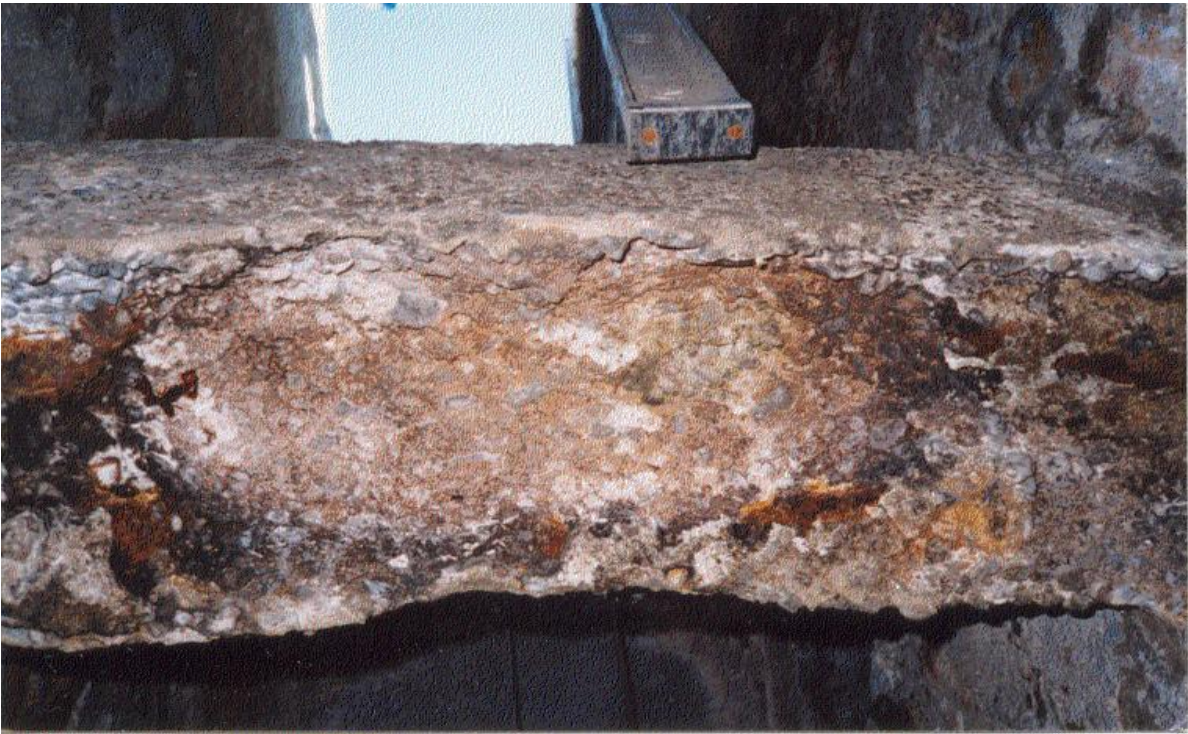
Figure 2. Lift Station Prior to Rehabilitation.
