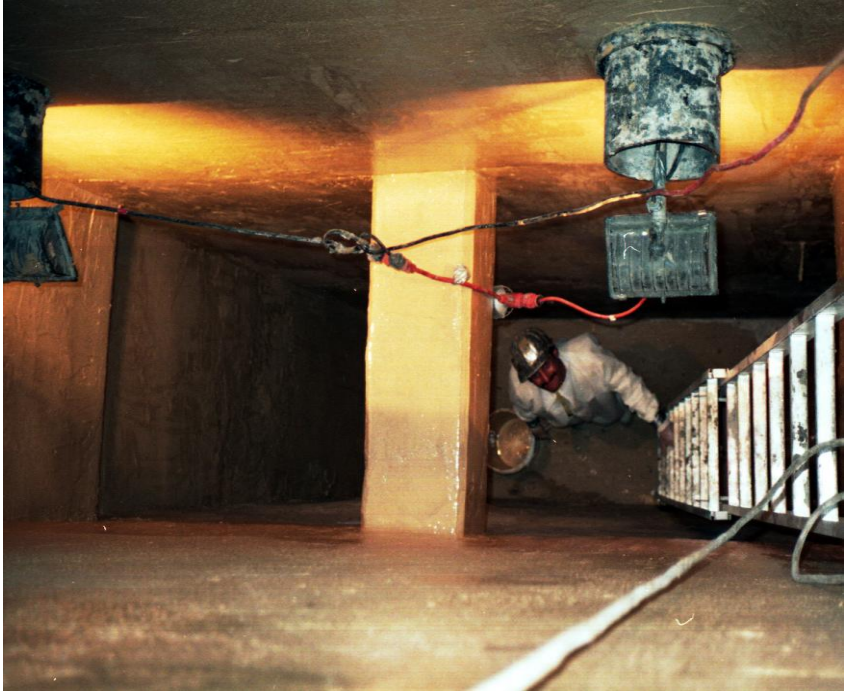
Figure 5. Rehabilitated Lift Station.
