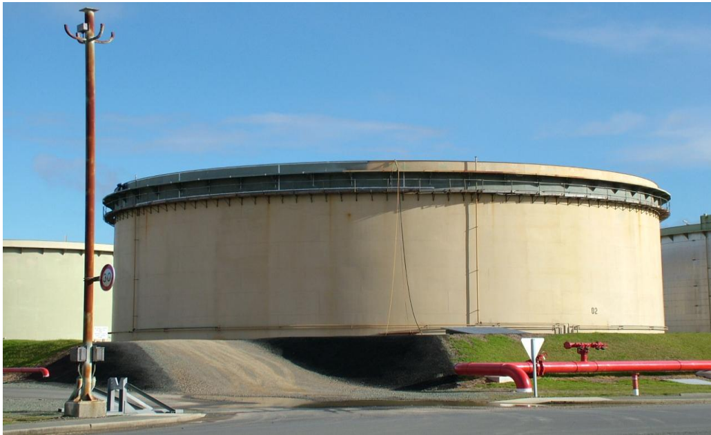
Figure 1 Exterior View of Crude Oil Storage Tank
