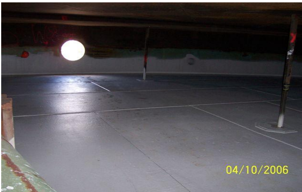
Figure 5 Completed Lining
