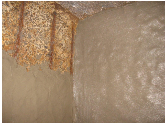
Troweled applied underlayment at ½ inch
