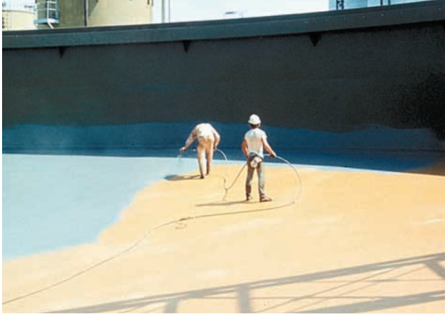
Addition of an optional topcoat provides further defense against permeability.
