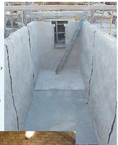
Refractories backed by a membrane are ideal for hot, acidic environments.
