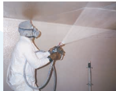
Fiber-reinforcement adds to the durability of Sauereisen linings.
