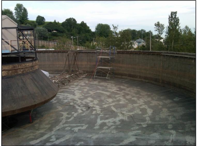
After the epoxy pour & spread sand mixture was allowed to cure overnight, the excess sand was swept from the surface and collected for use on adjacent area on the other side of the rake arms.
