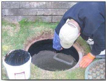
Manhole ChimneySeal is easily applied by gloved hand (neoprene or rubber). The most practical method of applying the product within small diameter structures is to wipe the material on with a gloved hand. Application by spatula or trowel is also acceptable.
