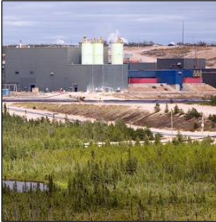
Key Lake Uranium Processing Facility
