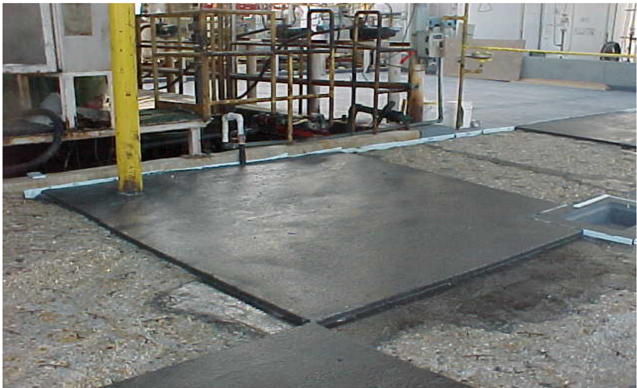
New off-loading pad at a sulfuric acid processing area
