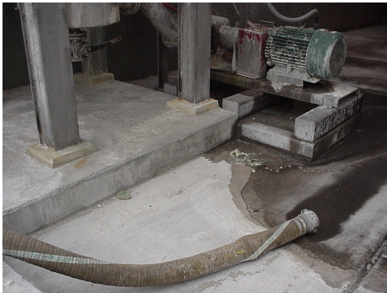
Tank pad & pump base poured with polymer concrete
