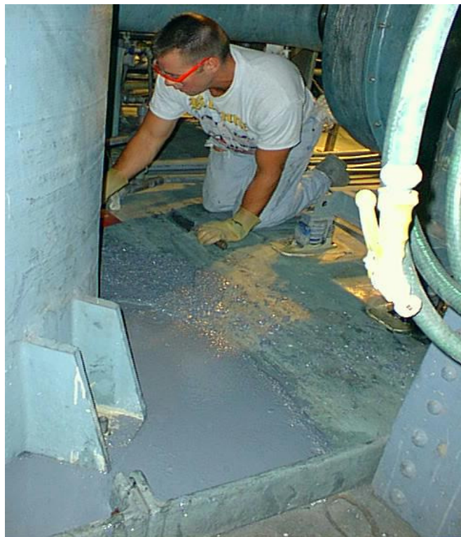
Concrete pad rehabilitation with polymer concrete around a sulfuric acid tank
