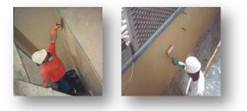
Each formulation of SewerGard provides an impermeable, high strength, corrosion-resistant lining for structures subject to infiltration and attack from hydrogen sulfide and acid generated by microbiological sources.
