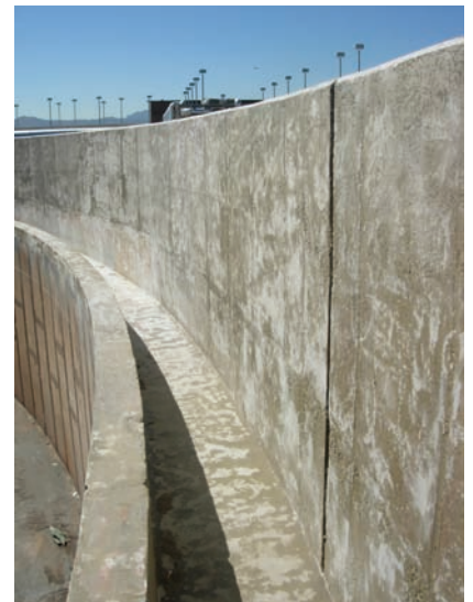
Condition of structure following re-surfacing with a light-weight epoxy underlayment.
