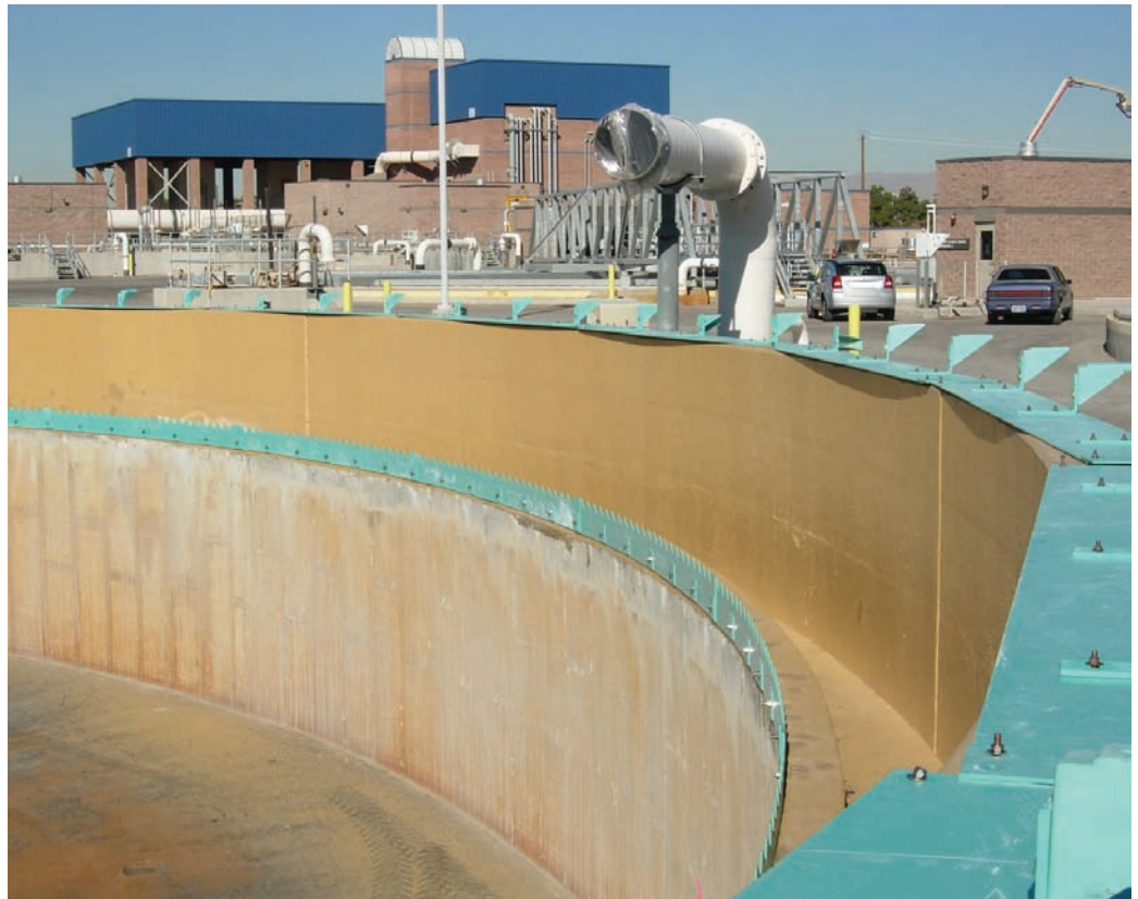
Applicators applied 125-mils of the SewerGard epoxy lining.
