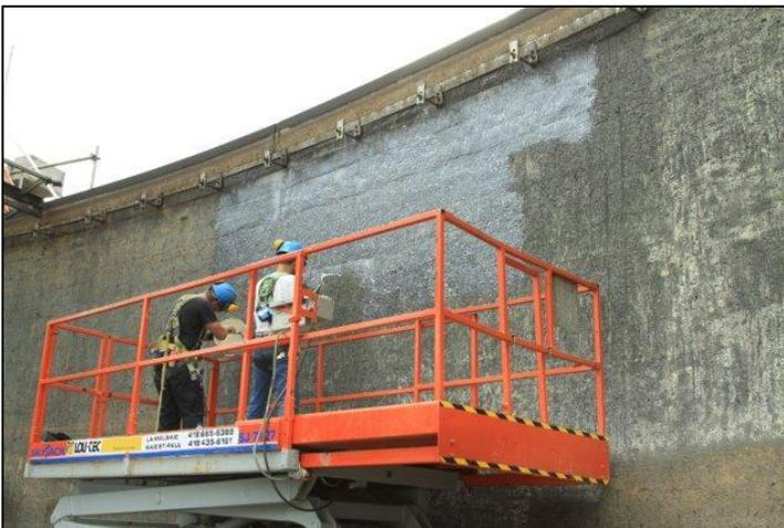
The epoxy repair mortar is specifically formulated to bond to rough concrete surfaces with the ability to fill imperfections and bug holes without sagging or outgassing. Not only does the concrete surface get refinished to an acceptable surface for application of the lining; but, the epoxy concrete repair material does not require a primer and offers a 72- hour recoat time for coordination of your lining or coating application.
