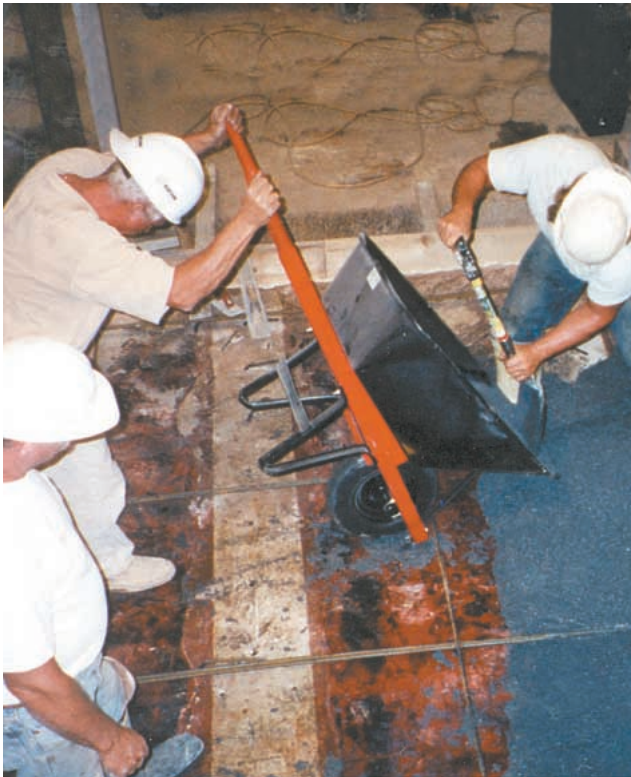
Polymer concretes exhibit working properties and application methods similar to standard Portland-based materials.
