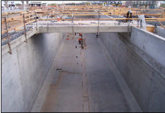
Chambers prior to sandblasting
