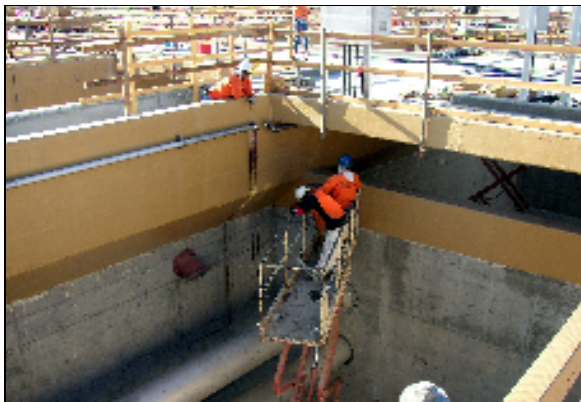
Lining touch-up following spark testing
