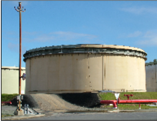
Crude Oil Tank
