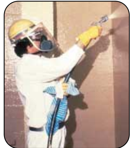
Spray installation is the quickest method for new construction or maintenance.
