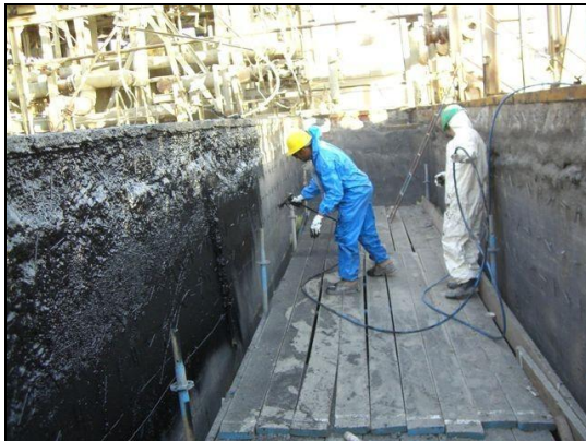
Spray Application of No. 89
