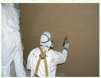
**SewerGard® 210S - Sprayable** is fiber-reinforced for a high degree of durability. 210S allows quick Installation in a single 60 mil coat when applied by standard airless equipment. It is ideal for large-scale applications.
