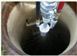
**SewerGard® 210FS - Fast-Set** is a fast-setting epoxy material engineered for the protection of manhole benches, inverts and other structures which are subject to very little maintenance downtime. Also available in ultra-fast-setting version.
