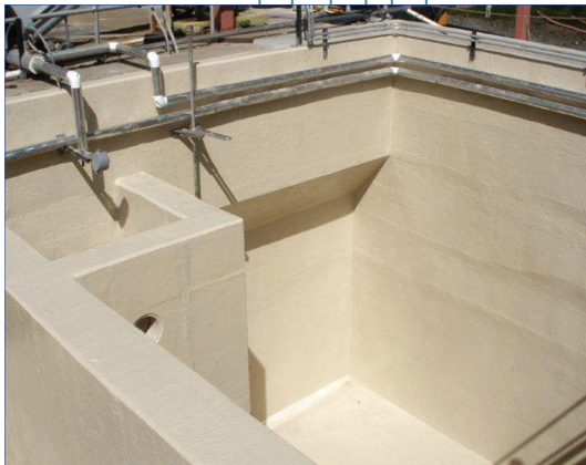
SewerGard® 210X applied in a digester
