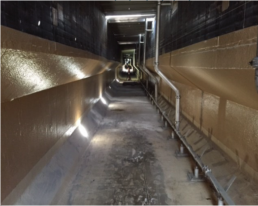
SewerGard® 210S in an influent channel
