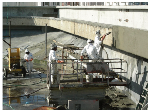
RestoKrete® F-121 applied by shotcrete
