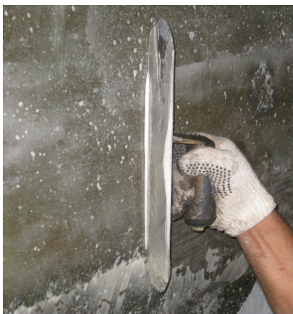
Bughole filling with RestoKrete® 209
