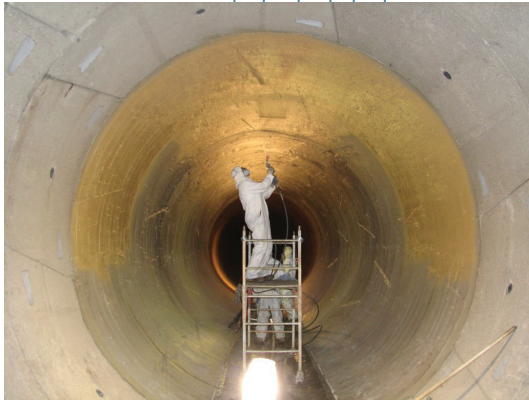
SewerGard® 210S applied in a tunnel
